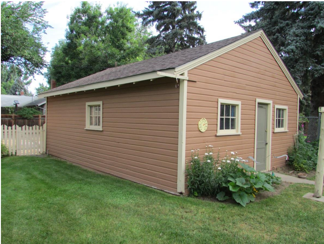
South and West Elevations, Two-car Garage built 1968, July 2014
