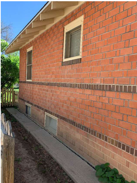
Rear bathroom & NW window on west elevation
