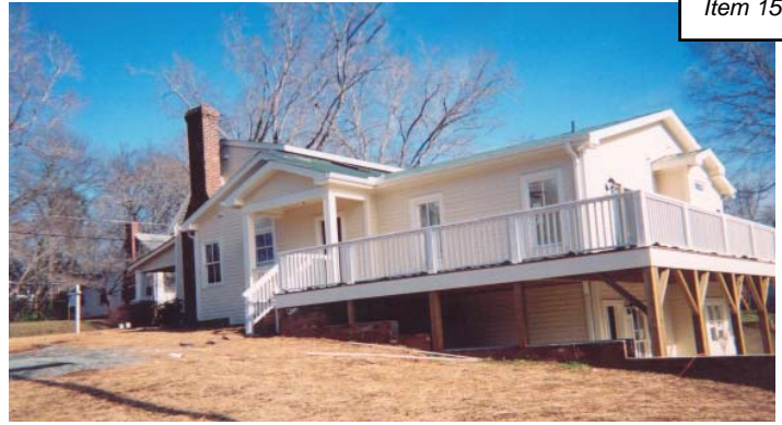
The size of this new rear addition—incorporating two floors and an extended depth—combined with substantial changes to the site overwhelm the modest historic house.
