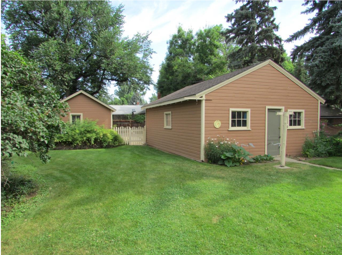
Garages facing North, July 2014
