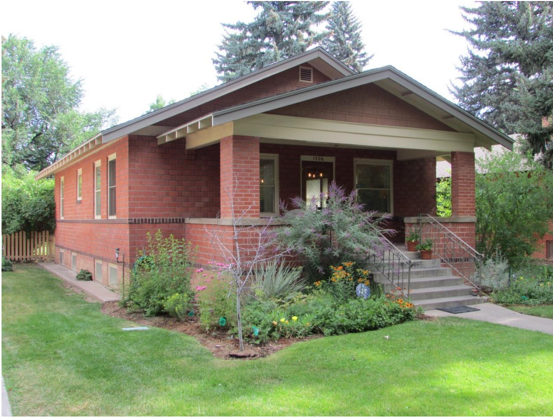
Front (South) and Side (West) Elevations, July 2014
