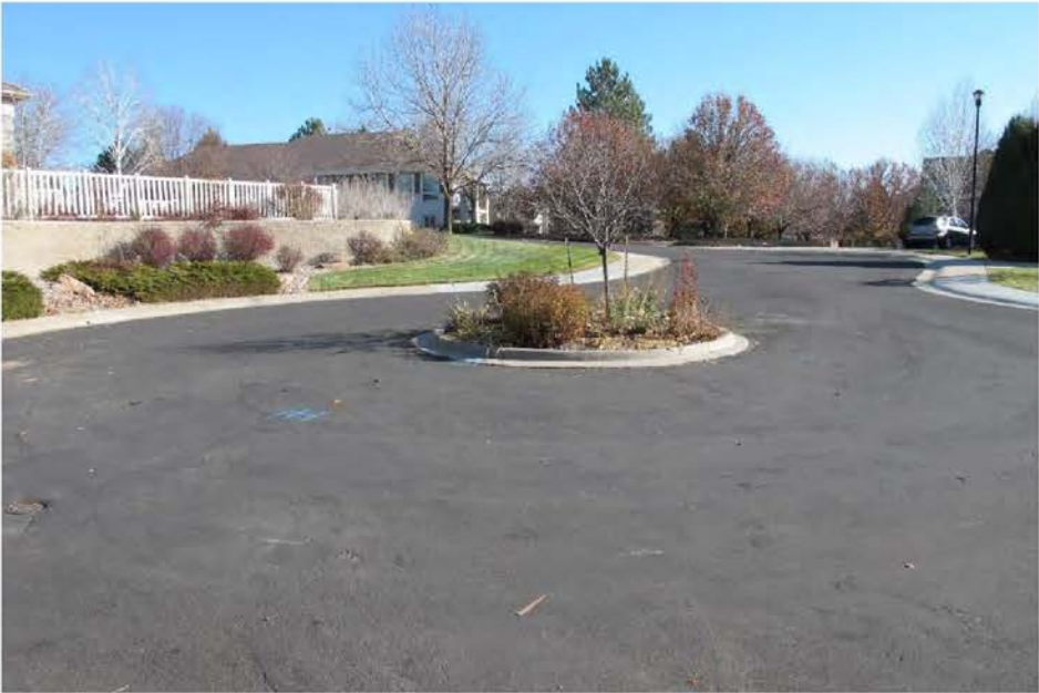
Existing pavement / Viewing east on east-west portion of Castle Ridge Place
