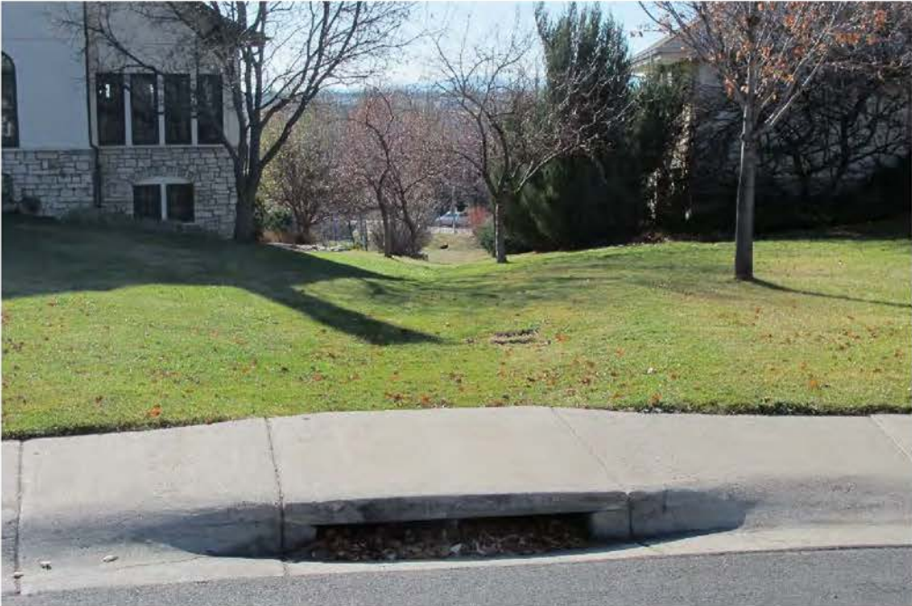
Sidewalk culvert at low point of Castle Ridge Court cul-de-sac pond outfall pipe in far background
