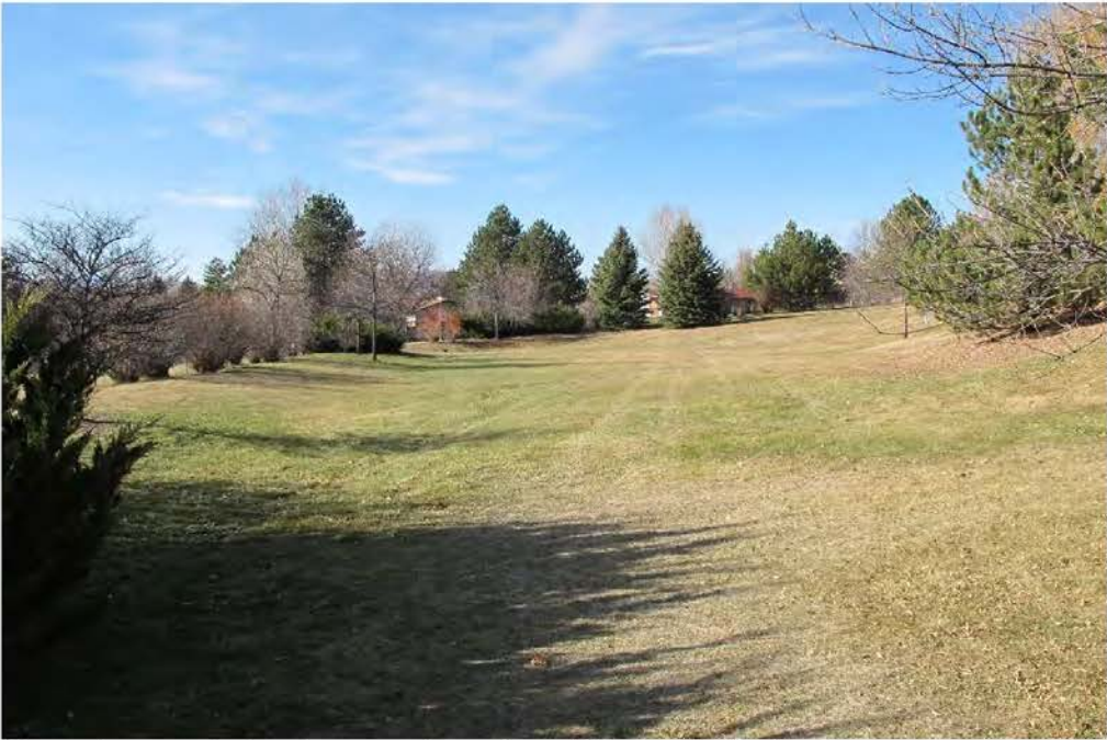
Detention pond viewing west / pond outfall pipe in far background
