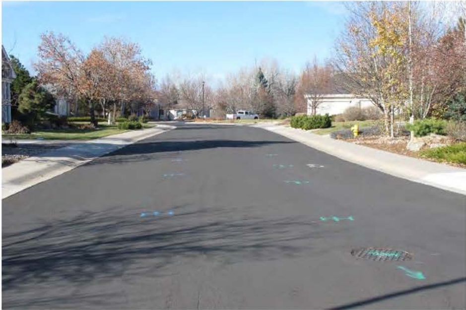
Viewing west on east-west portion of Castle Ridge Court
